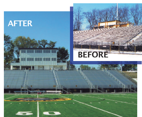
Existing Structure Renovations
