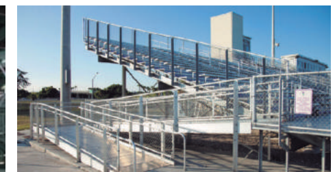
Ramped ADA Access
