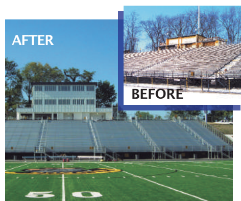
Existing Structure Renovations
