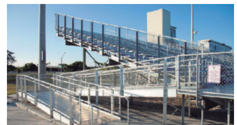
Ramped ADA Access
